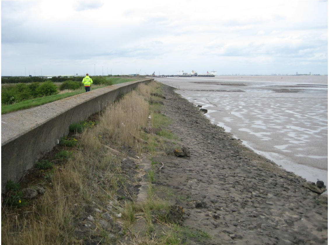
Figure 2-1: Photograph of the typical tidal flood defences in the Humber region
